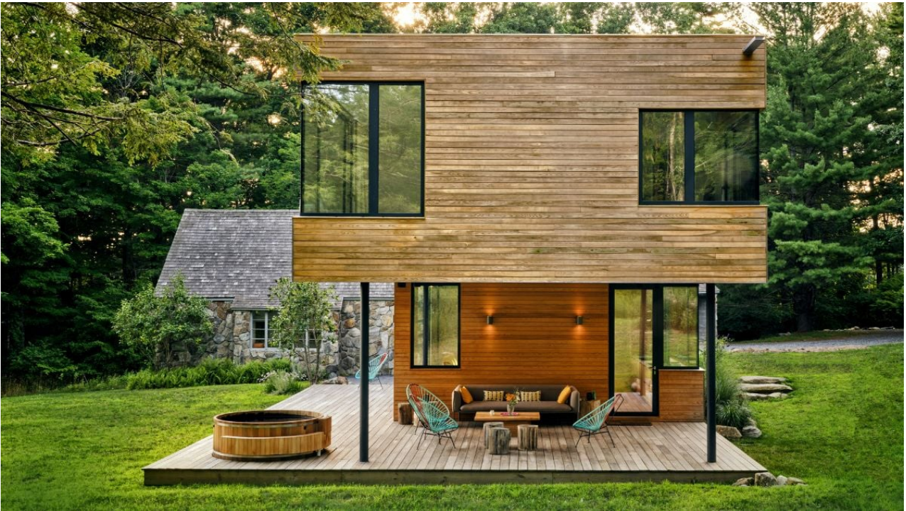
The two huge corner windows, one off each bedroom, that blur the distinctions between indoors and out are the showpiece of the modern addition, which is clad in horizontal cypress siding.
