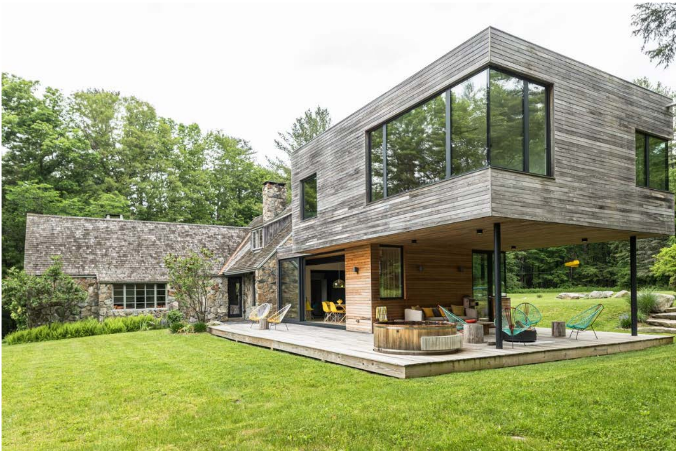
Ms. Jefferys designed the second floor to cantilever off the first floor, creating a covered porch below. JULIE BIDWELL FOR THE WALL STREET JOURNAL
